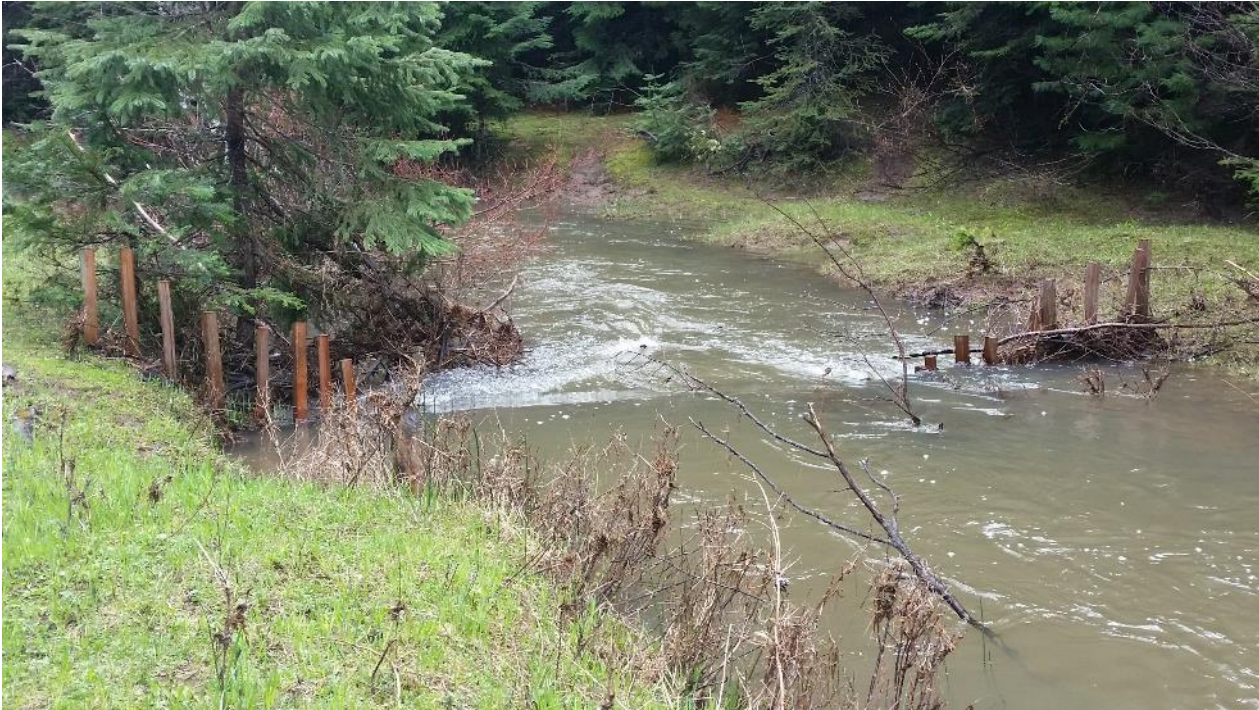
Figure 3. FBD on Corral Creek during receding flood flow.
